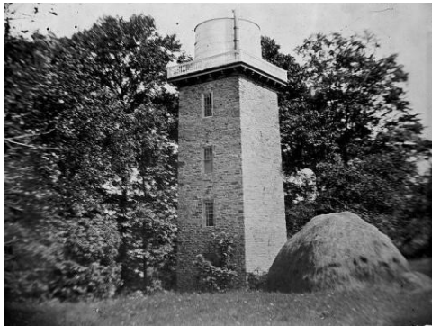
1800s Glen Foerd Water Tower
