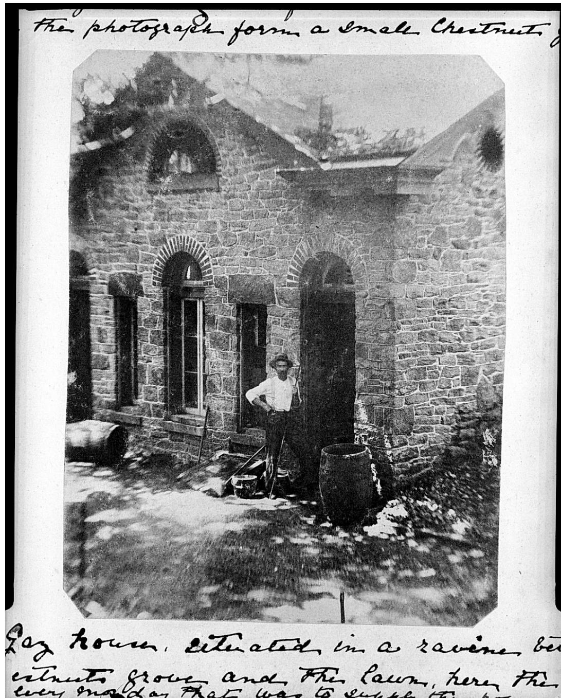
Gas House before conversion to cottage, n.d. (Macalester period). Macalester album reproductions, Glen Foerd collection.
