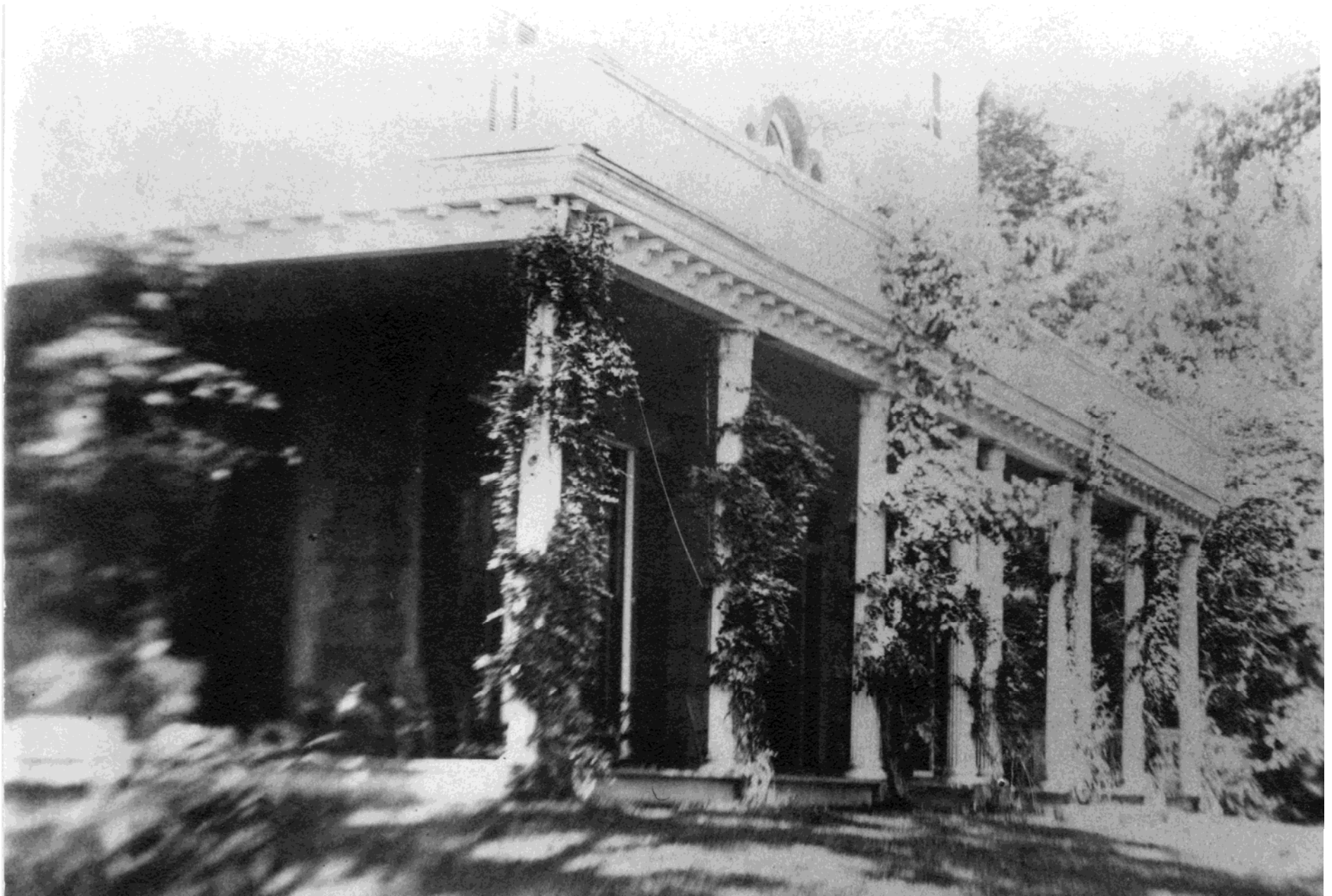
Detail, view of southeast side of building, looking northeast, n.d. (Macalester period). Macalester album reproductions, Glen Foerd collection.
